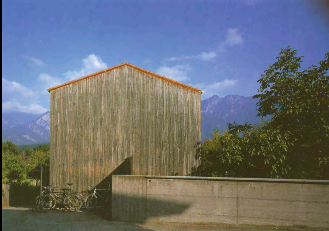
Original Studio and Office, 1985-86
